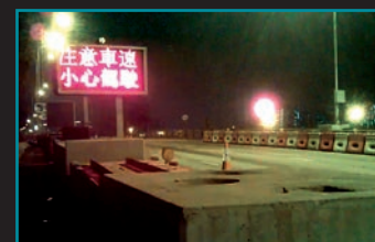
Installation of speed detection variable message sign 安裝測速顯示屏
