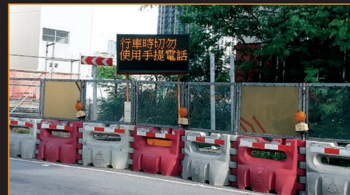
Installation of remote control variable message sign 安裝無線控制顯示屏
