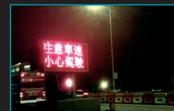
Installation of speed detection variable message sign 安裝測速顯示屏
